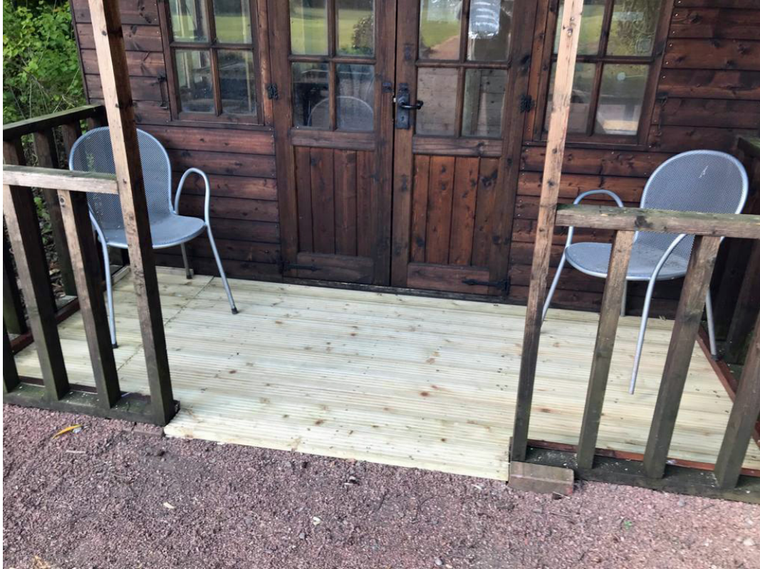
Repaired flooring at chateau on 1 st Tee.
