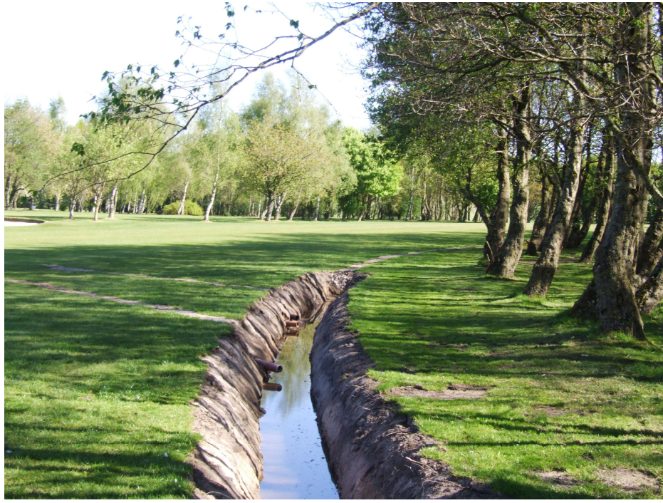
New ditch at right hand side of 2 nd .
